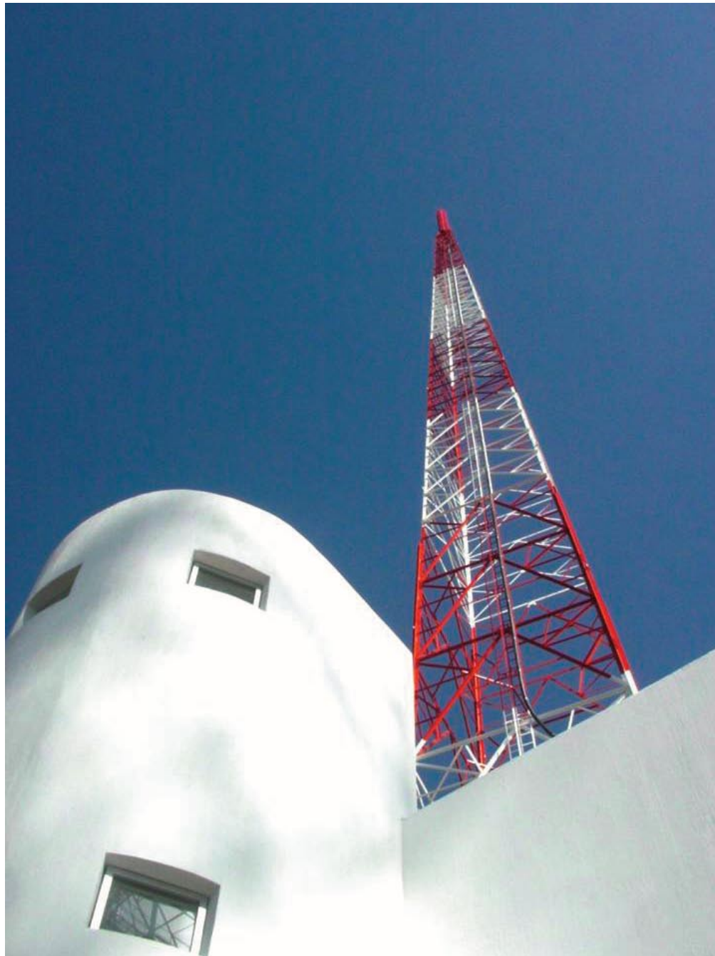
Channel 44 Transmissions antena.
